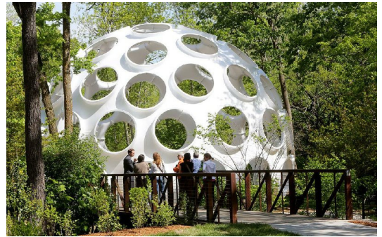
R. Buckminster Fuller (1895 - 1983) Fly's Eye Dome , 1961, fabricated ca. 1980 Fiberglass-reinforced polyester, 38 × 50 × 50ft. Crystal Bridges Museum of American Art, Bentonville, Arkansas, 2015.15
